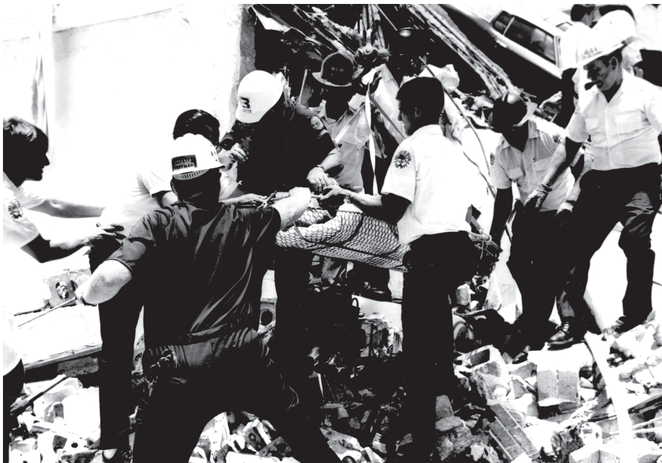
Rescue workers take injured victims from the DEA Miami Office Building following its collapse on August 5, 1974.
