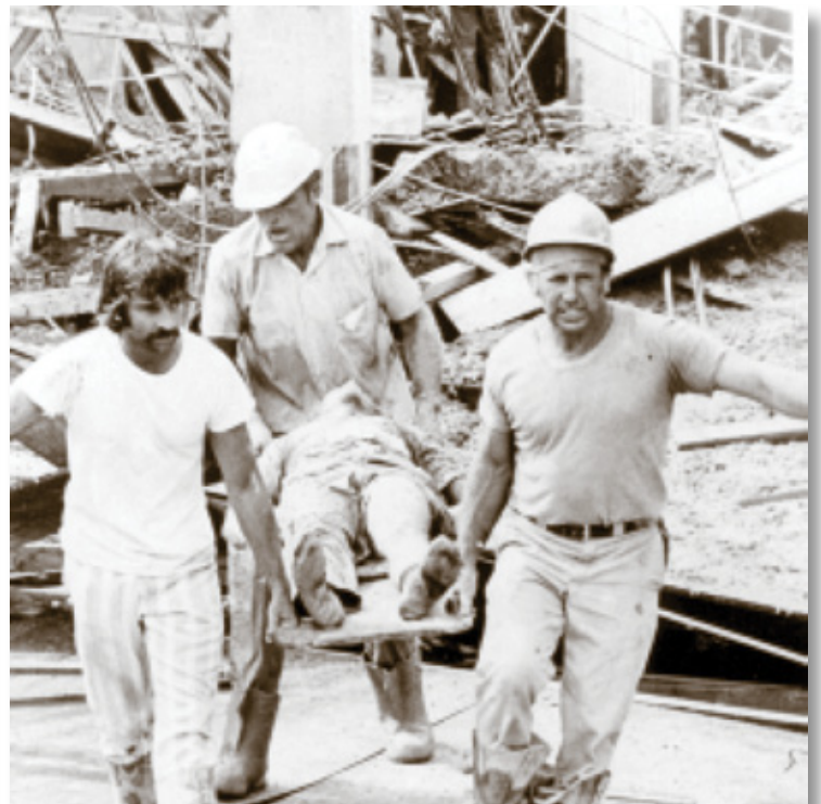
Rescue workers take injured victims from the DEA Miami Office Building following its collapse on August 5, 1974.
